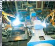
Main frame welding line
