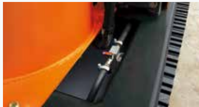
Fuel tank water drainage cock
